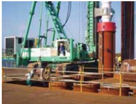
Photo 2 Driving of steel pipe piles
