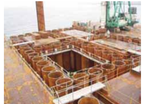
Photo 3 Construction of steel pipe sheet pile well foundation
