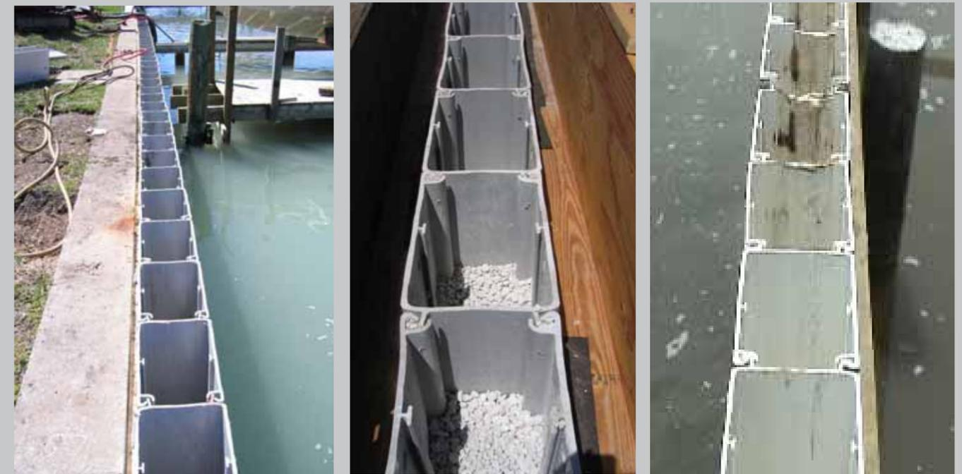
**The Series 800 plastic piles provide a section modulus of 892.5 cm<sup>3</sup>/m and a Bending Moment of 19.7kNm/m!**
