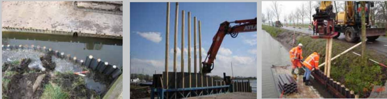
**MultiLock uses up to 2 x 100mm diameter posts or tubes**
