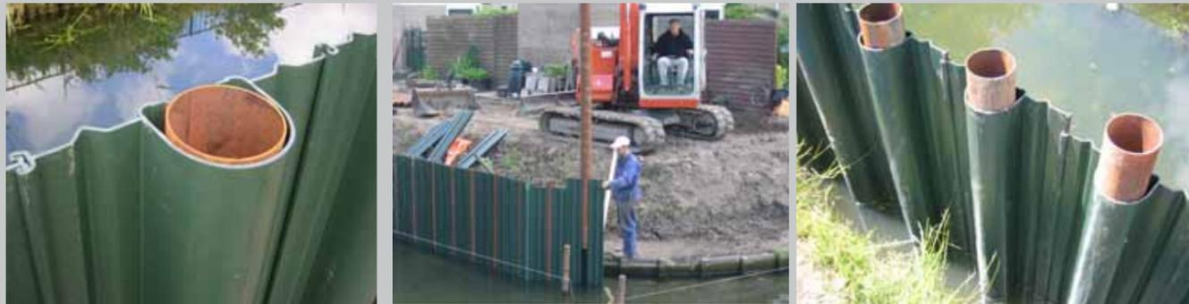
**Piles get their strength from the material and their cross sectional shape. PVC will never have the strength of steel, so plastic piles need new designs. Only APE offers these - all others replicate the shape of steel piles.**
