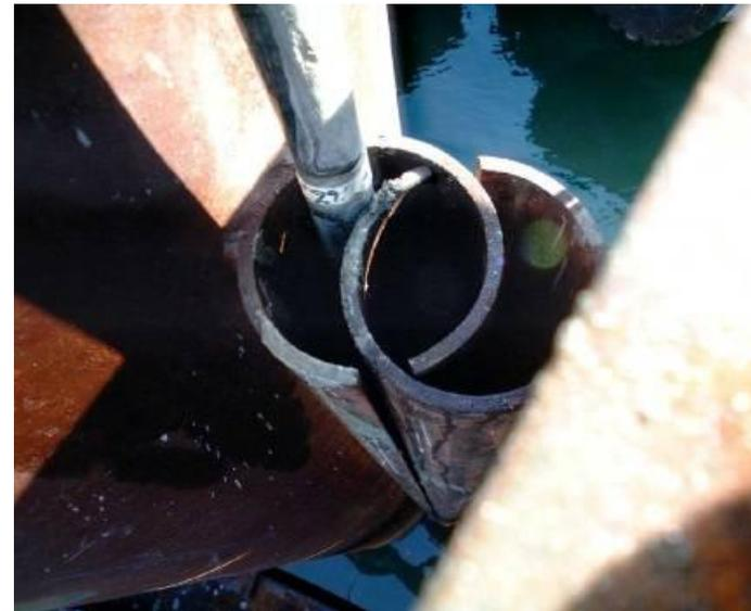
.-2) Fill joint pipes with mortar
