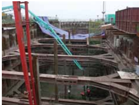
Photo 6 Interior of well foundation
