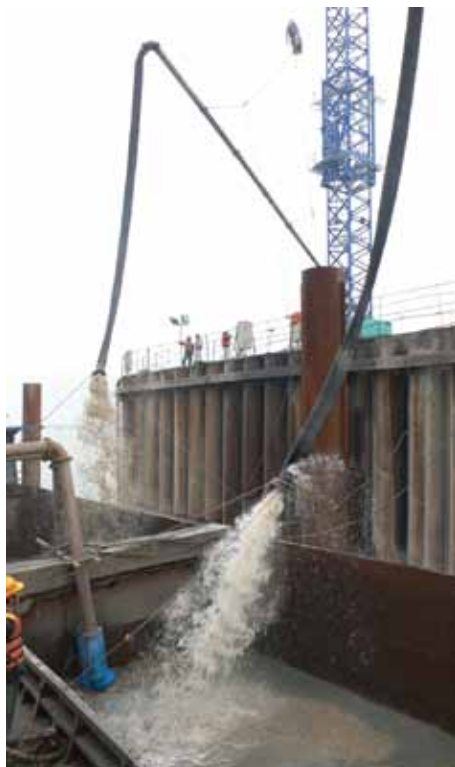
Photo 7 Discharge hole of underwater drilling pump
