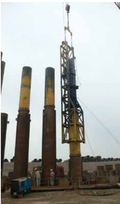
Photo 5 Final driving of steel pipe piles using diesel hammer
